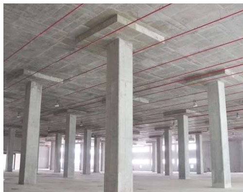
Fig 2: Flat Slab Drop panel in Building
