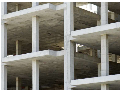
Fig 1: Simple Flat slab
