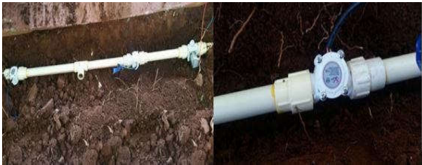
Fig.4: Water flow sensor placement
